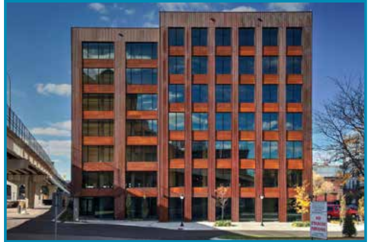
T3 Tower, a seven-story high rise in Minneapolis, MN, was the first modern tall wood building constructed in the US. Source: https://www.architectmagazine.com
